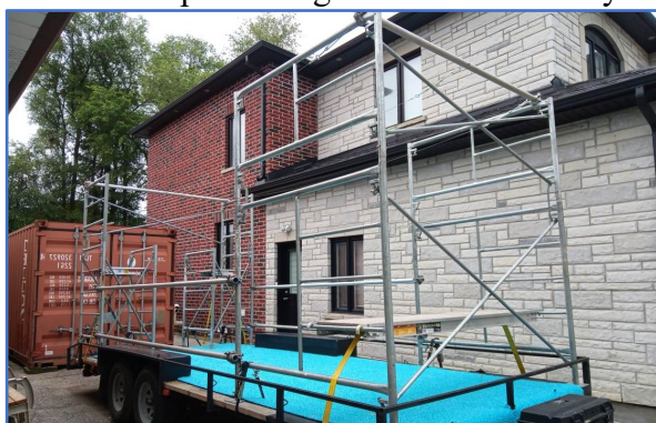
Fig. 1 Initial assemble at the home of the author (RKNS)
